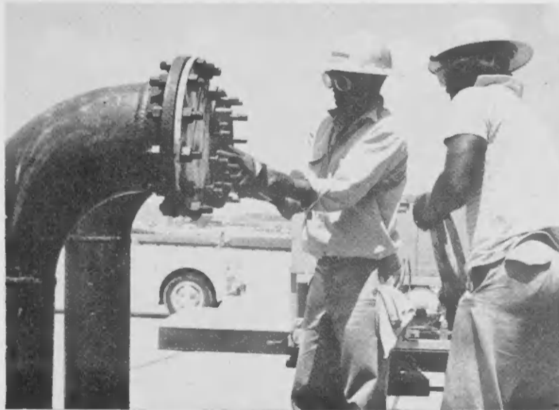
THE TWO men who connected the lines to the ammonia carrier were Calvin Schmidt and Adriaan Wever. Pumping ammonia aboard the Esso Centro America actually began at about 5:30 p.m., Aug. 3. Moments after the pumping had been started, the pipes, above, turned white with frost caused by the extremely low temperatures which keep ammonia in a liquid state. In sixteen hours, 4000 tons of Aruba ammonia were loaded aboard the carrier.
